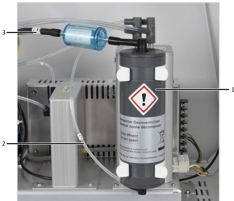
Fig. 70 Replacing the chemical ozone decomposer
